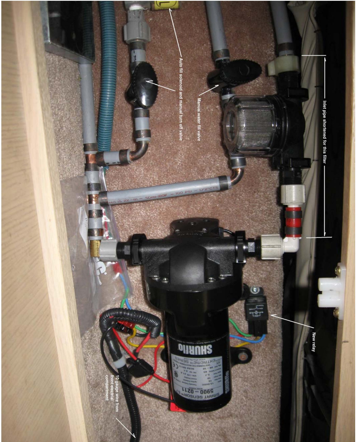
New pump installation with relay:
